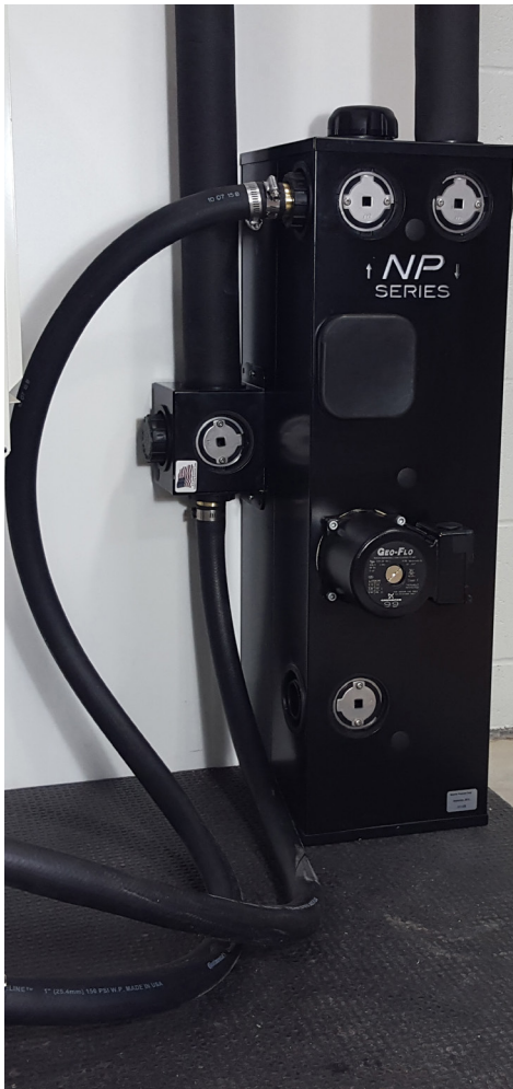
Figure 7: Flow center mounted 3-way valve
