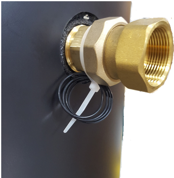
Figure 5. O-rings zip-tied to upper right connection on tank
